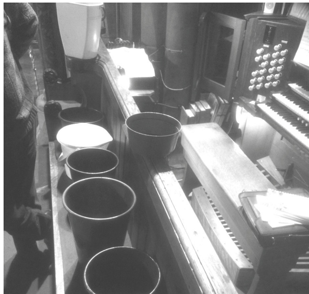
ABOVE: Buckets ready in St Paul's. Storm Doris wasn't helpful to two of our churches, even though the insurers refer to her as "an act of God!" Church roofs suffered damage at St Paul's and St David's (report from St David's below)
